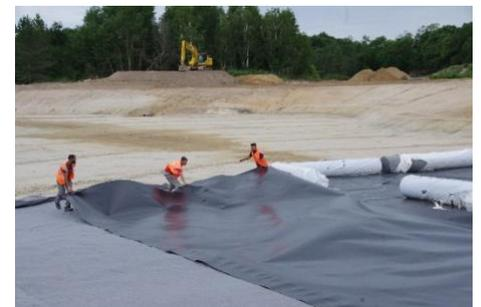
*Installation of the ST300 puncture-resistant geotextile and HDPE*
