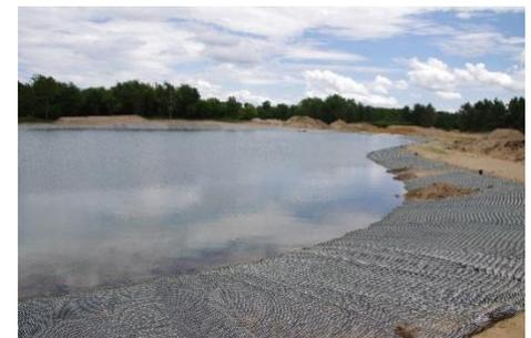
*Installation of soil retention netting and backfilling*
