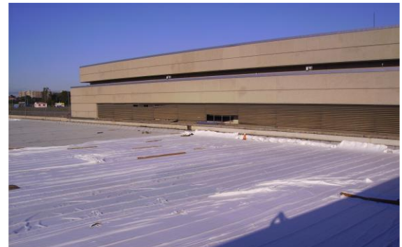
DRAINTUBE® installation on the subgrade
