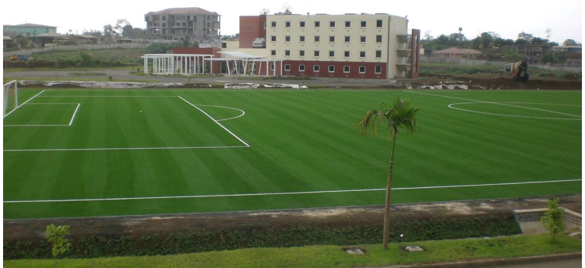
FIFA quality soccer field construction – Malabo – 2009
