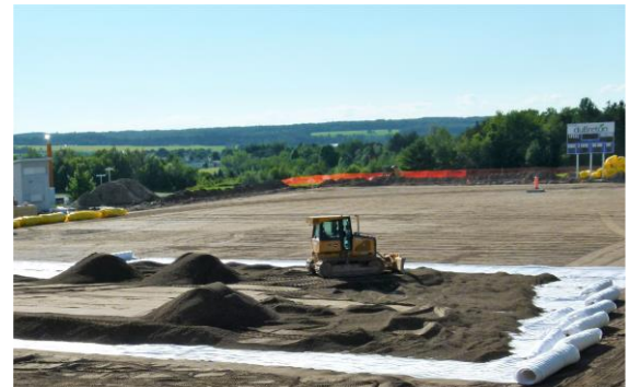
Backfill placement on the DRAINTUBE®
