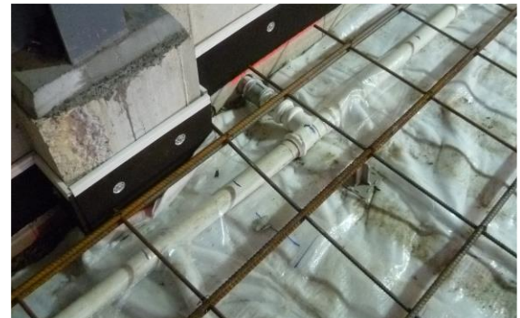
Connection of the DRAINTUBE® to the collector pipe using Quick Connect system for active SSD.
