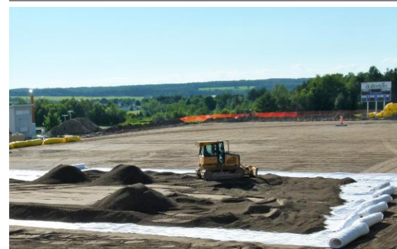
Backfill placement on the DRAINTUBE®.
