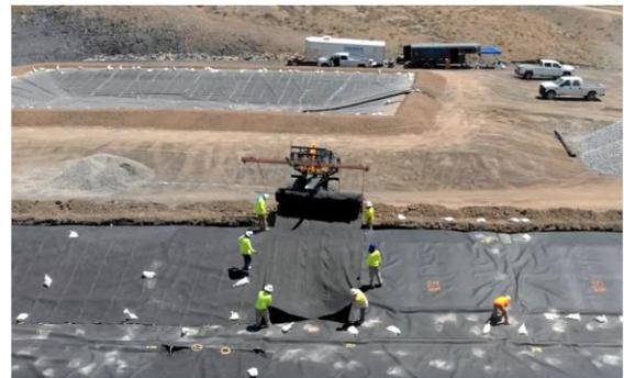
Installation in the slopes using a spreader bar. When the use of such equipment is possible, the installation is even faster.
