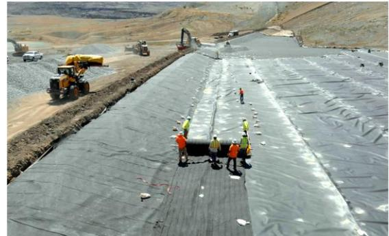
Manual installation of DRAINTUBE 606 ST1 D20 as part of the leachate collection system over a 60-mil HDPE geomembrane. Light rolls are easier and faster to install.
