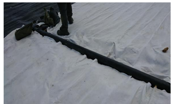
Mechanical connection of the DRAINTUBE mini-pipes to the header pipe using Quick Connect system.
