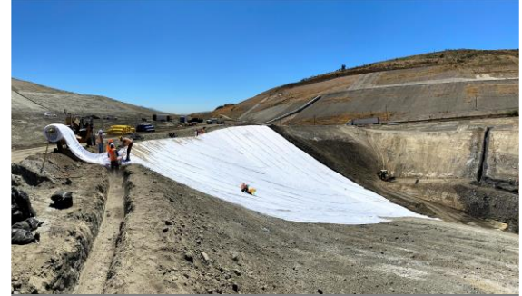
Installation of DRAINTUBE 303P FT4 D25 for gas venting below the liner. Each DRAINTUBE® panel is connected to the next one using Couplers.
