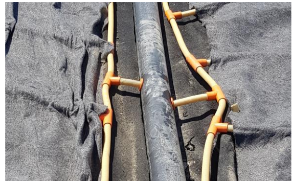
The Quick Connect System technology is used to reduce the air intrusion and allow a gas extraction with a vacuum.
