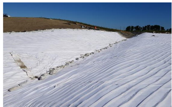
DRAINTUBE 500P FT4 D25 is installed above the liner for surface water drainage as well as protection against puncture.
