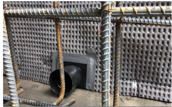
T-connector connected to the Soldrain 4000 to evacuate the water drained by the ALVEODRAIN EV to the outlets.
