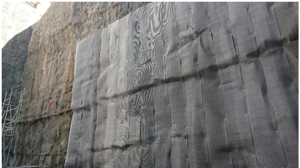
Vertical drainage of the Côte-Vertu garage walls - 2018
