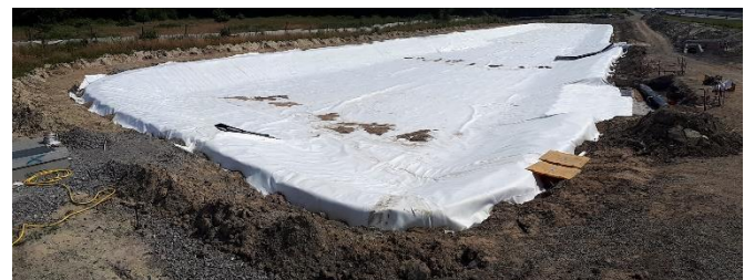
Installation du géotextile anti-poinçonnant
