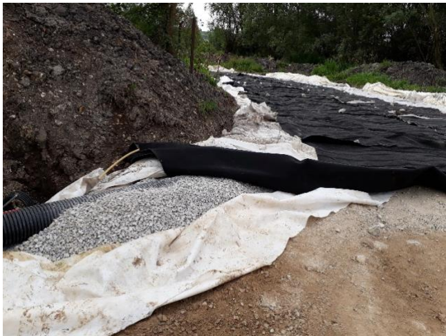
Connection to the collector trench
