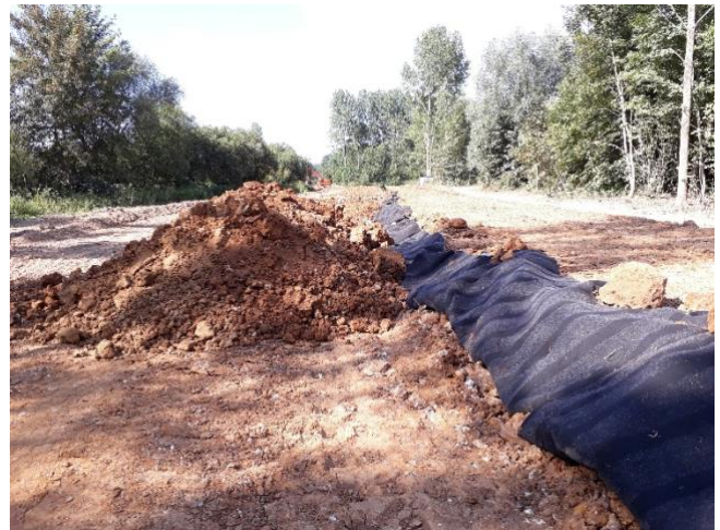
Vertical installation of DRAINATEX ("concertina-like")
