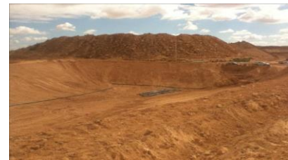
Figure 2: Excavation of basins
