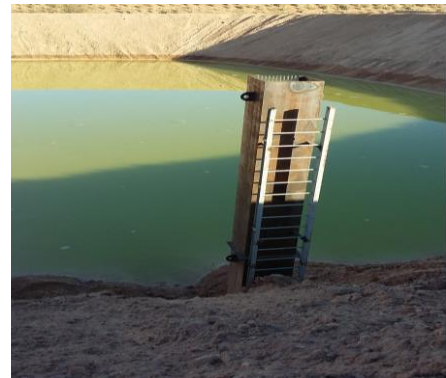
Figure 9: Control basin recovery chimney.
