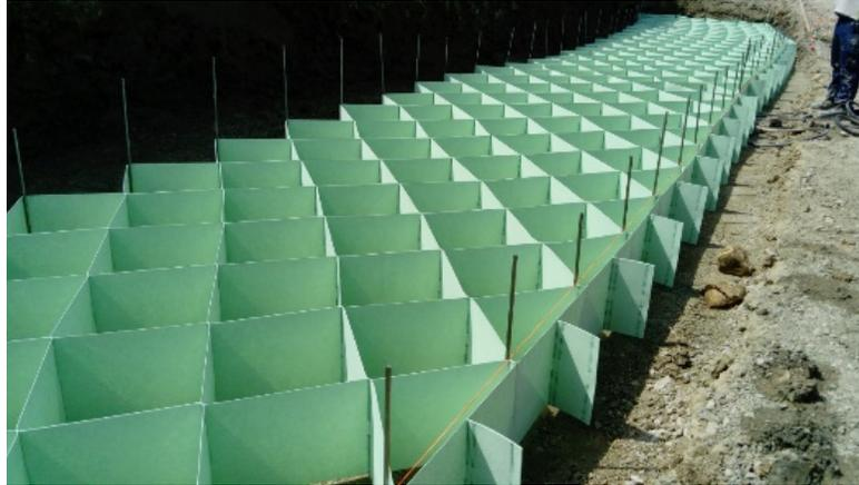
**Figure 10. Geocells deployment.**
