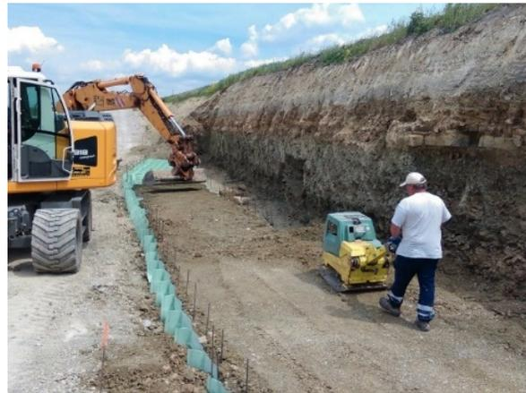
**Figure 11. Backfilling and compaction.**
