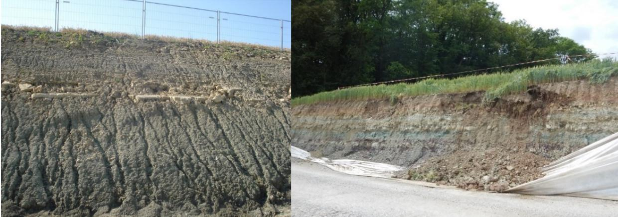
**Figure 2. Erosion on the slope and beginning of landslide.**
