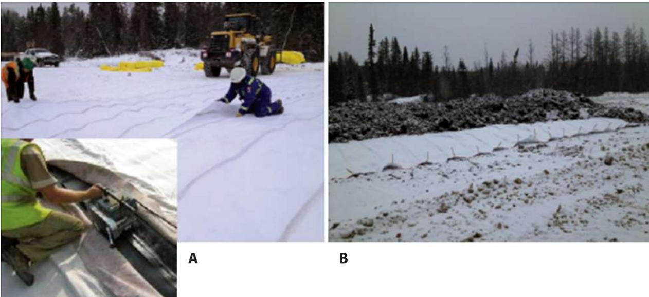
**FIG 4** – Central Manitoba Mine (Canada) abandoned tailing rehabilitation site: (A) deployment and installation of DRAINTUBE™ ensuring overlap between drainage tube liners. Insert – sealing of drainage tube liner together; (B) deployed drainage tube liner with peat overlain.
