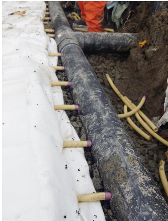
**Figure 3: Connection of the minitube blanket to the collector pipe.**
