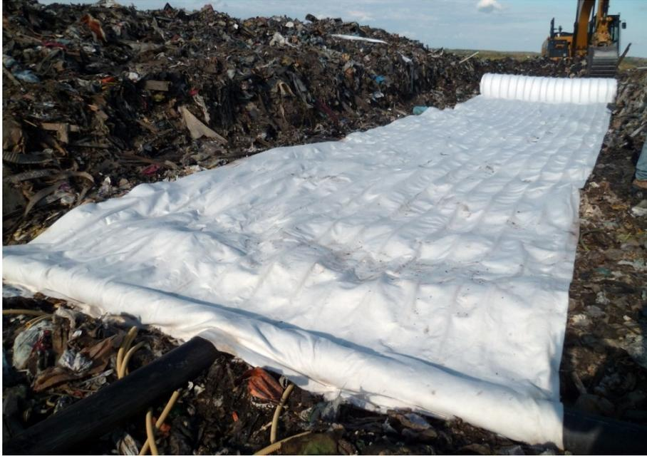
**Figure 2: Minitube blanket installation.**
