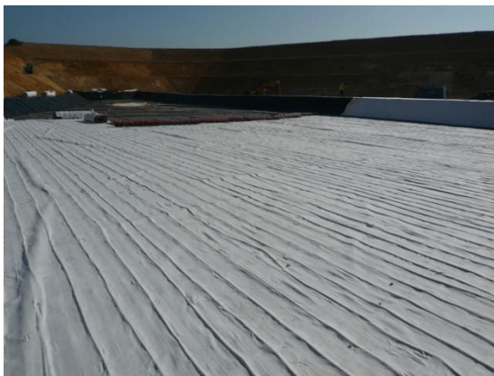
Figure 2. Leachate drainage at the bottom of land-fill
