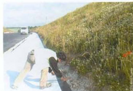
Photo 6 Fixation du Stabiliner Alveo Securing the Stabiliner Alveo
