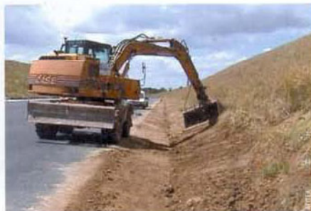
Photo 8 Léger compactage et profilage final Light compacting and final shaping
