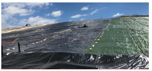
To further limit air intrusion into the gas network, DRAINTUBE® geocomposite can be manufactured with an associated coated woven polyethylene geomembrane on its upper side.
