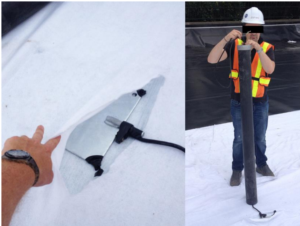
Figure 9: Example of a permanent access connected to the GEOCONDUCT®/DRAINTUBE® Conductive grid
