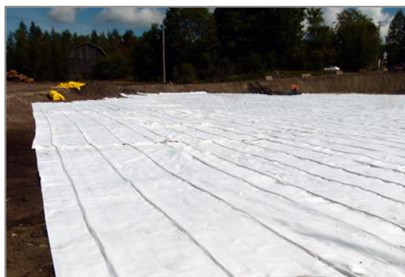
Figure 3: DRAINTUBE® installation
