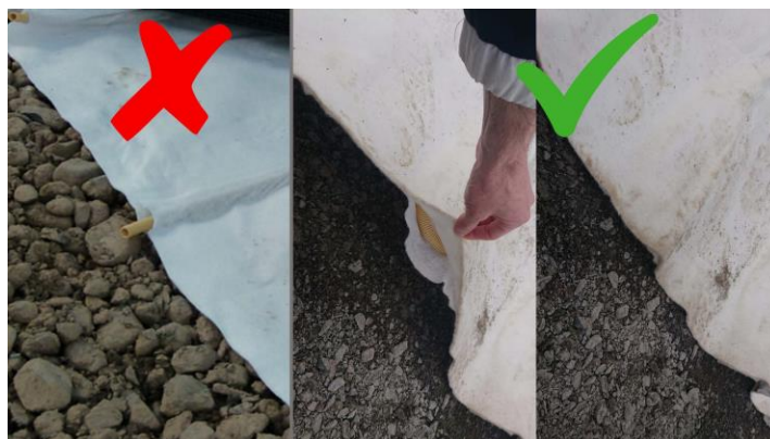
Figure 7: Mini-pipes between geotextiles
