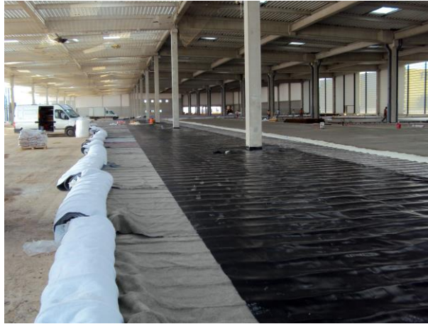
Figure 11: Casting of the concrete slab on the geomembrane
