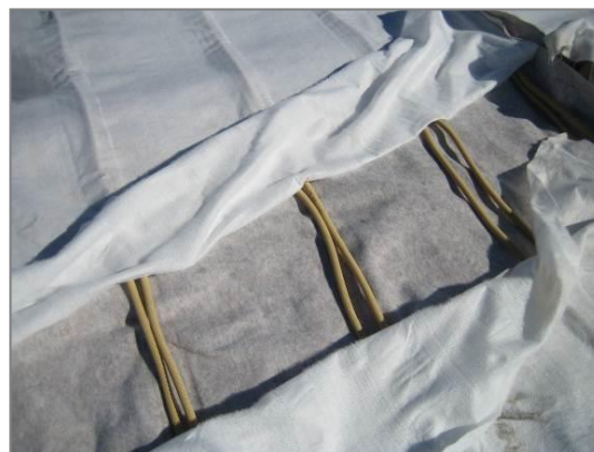
Figures 4: Transverse connections without couplers
