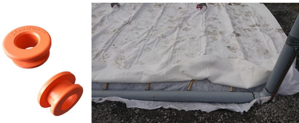
Figures 9: DRAINTUBE® connection to the collector pipe using the Quick Connect system
