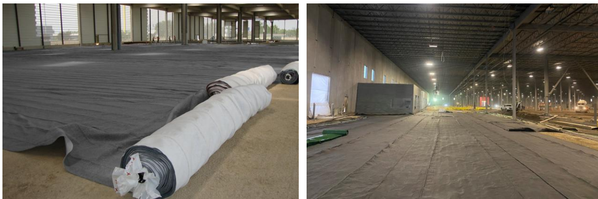
Figures 6: DRAINTUBE® installation on the subgrade
