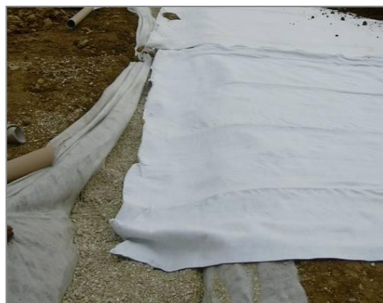
Figures 10: Connection to a collector trench
