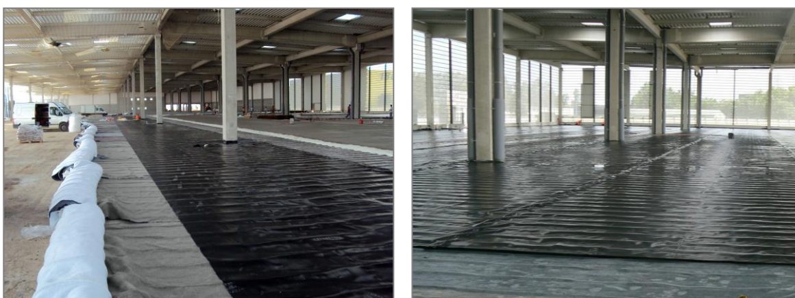
Figures 13: Upper geosynthetic layer placement
