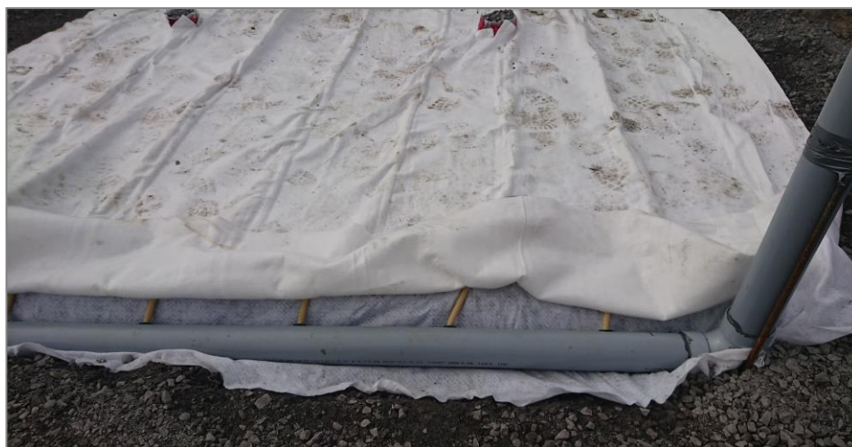
Figure 12: Connection to a plain drain with Quick Connect
