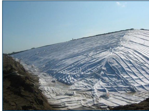
Figure 4: Installation du DRAINTUBE™
