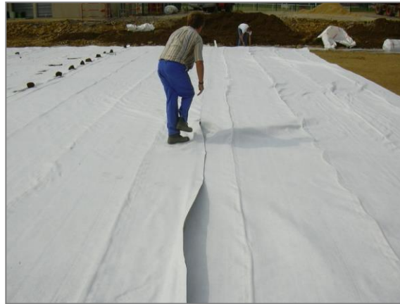
Figure 6: Side by side connections
