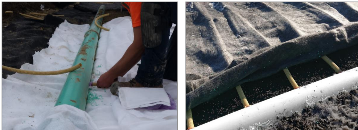
Figures 9: Connection to a solid collector drain with Quick Connects
