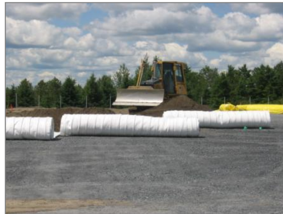
Figures 3: DRAINTUBE® installation
