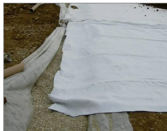
Figures 7: Connection to a collector trench
