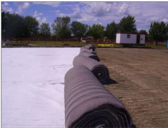
Figures 3: DRAINTUBE® installation
