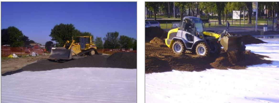
Figures 10: Backfilling
