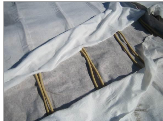
Figures 4: Transverse connections without couplers
