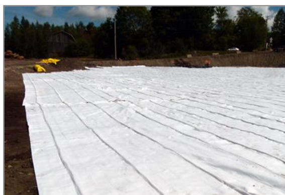
Figure 3: DRAINTUBE® installation
