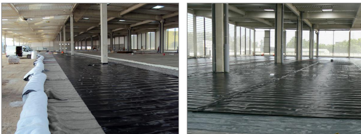
Figures 13: Upper geosynthetic layer placement
