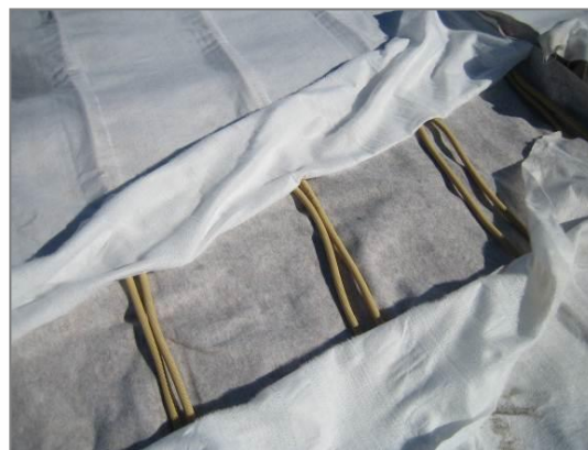
Figures 4: Transverse connections without couplers
