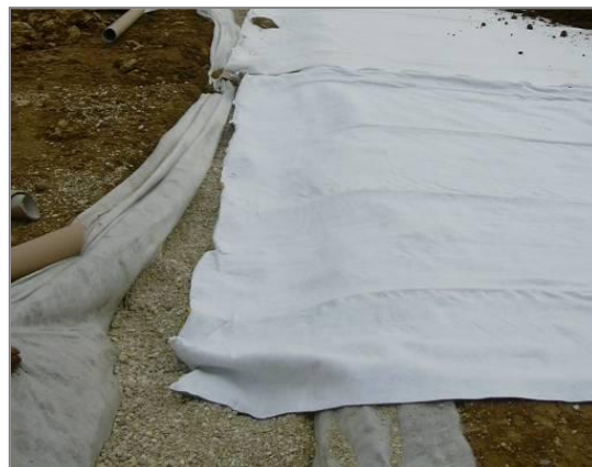
Figures 10: Connection to a collector trench
