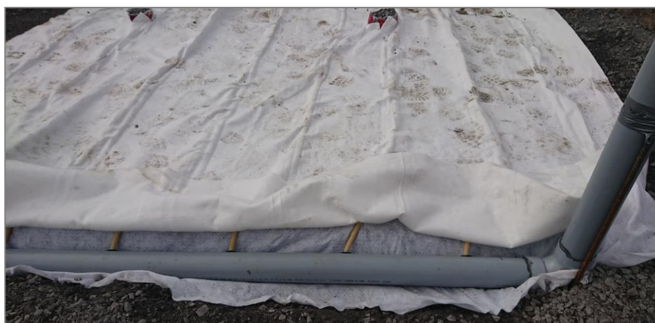
Figure 12: Connection to a plain drain with Quick Connect
