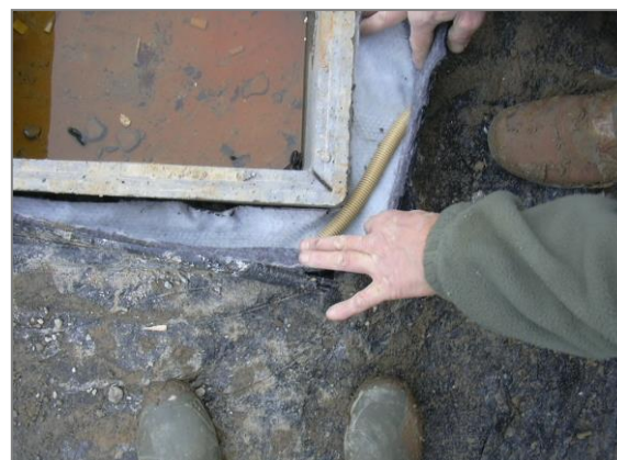
Figures 8: Passing of a narrow post
