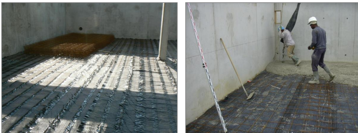
Figures 13: Pouring the concrete slab
