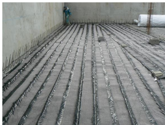
Figure 3: DRAINTUBE® FTB installation
