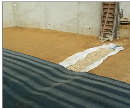
Figures 10: Connection to a collector trench
