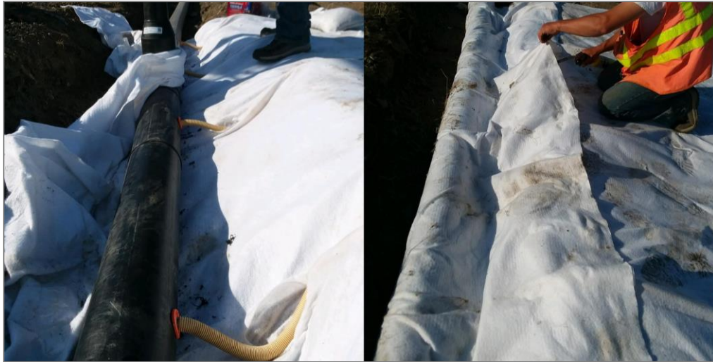
Figures 10: Connection to a plain drain with Quick Connect
