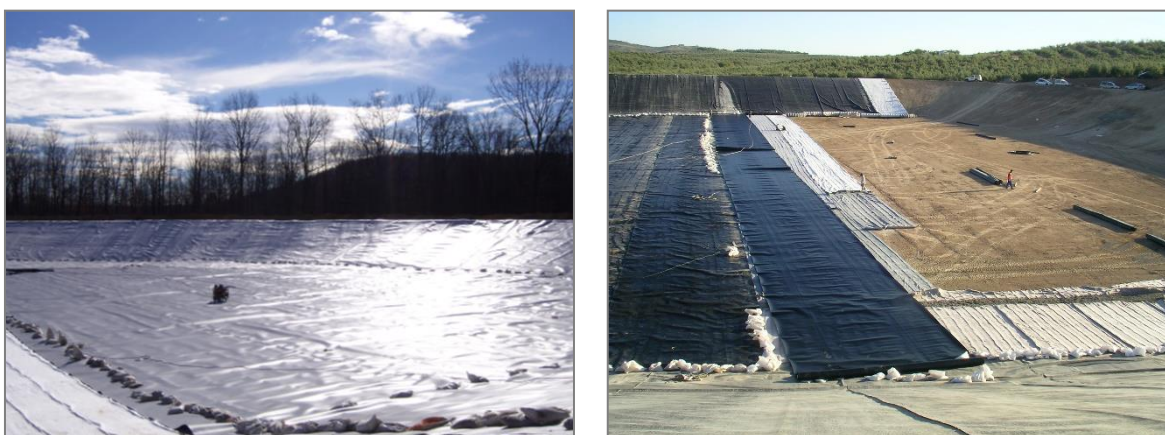
Figures 12: Geomembrane installation
