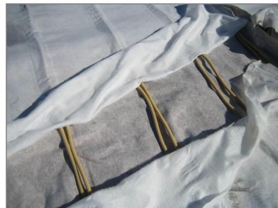
Figures 4: Transverse connections without couplers
