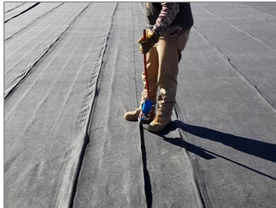
Figure 7: Side by side connections
