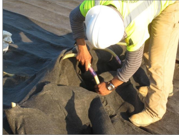
Figure 6: Mini-pipe junction with couplers
