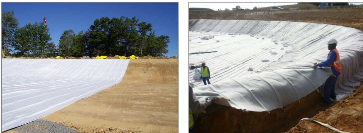
Figures 3: Putting into place of DRAINTUBE™
