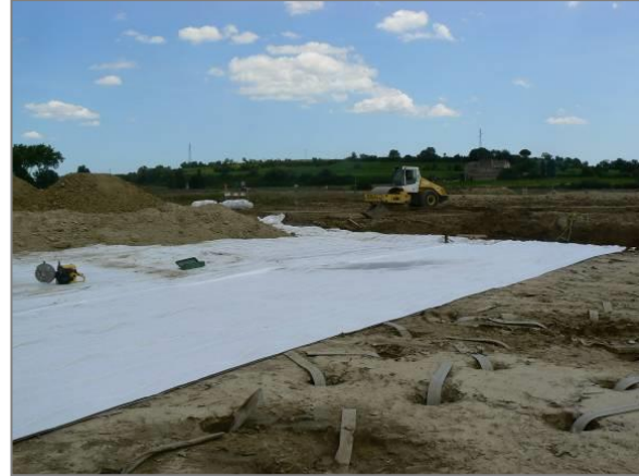
Figures 4: DRAINTUBE® placement over vertical wick drains
