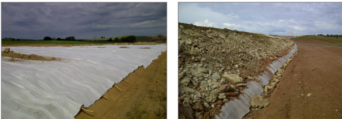
Figures 11: Termination in a ditch
