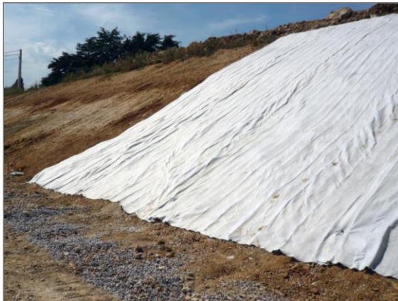
Figures 5: DRAINTUBE® installation on the slope
