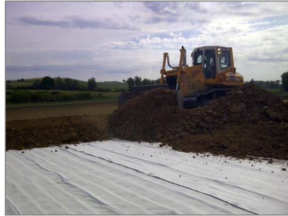
Figures 15: Backfilling - Embankment
