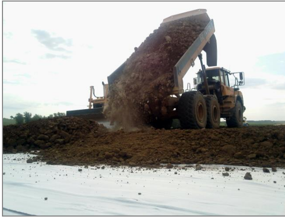
Figures 15: Backfilling - Embankment
