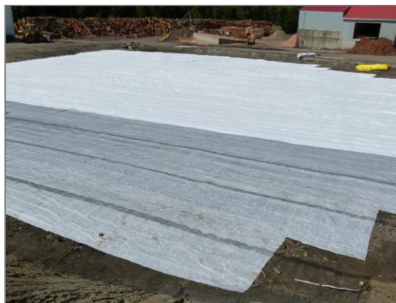
Figure 14: Upper geosynthetic layer placement
