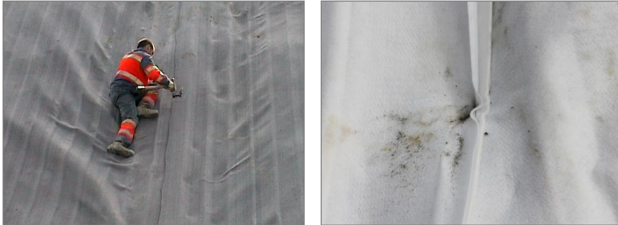
Figures 6: Mechanical fixations
