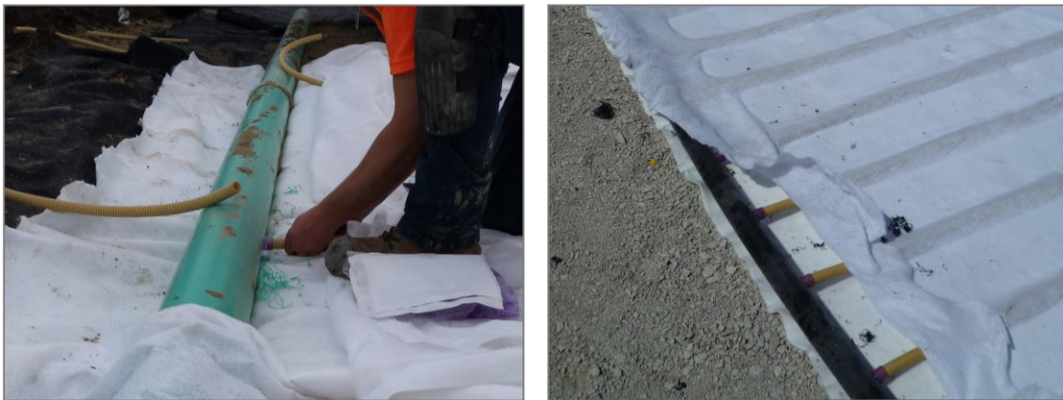
Figures 13: Connection to a plain drain with Quick Connect
