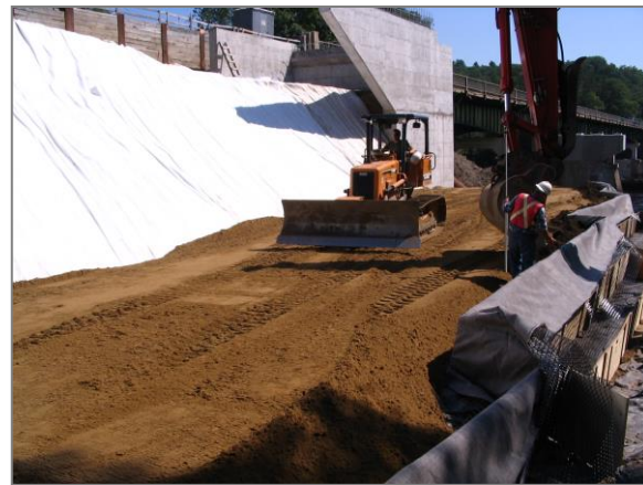
Figures 16: Backfilling – Draining mask and MSE wall
