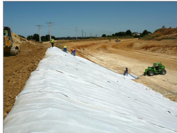
Figures 5: DRAINTUBE® installation on the slope
