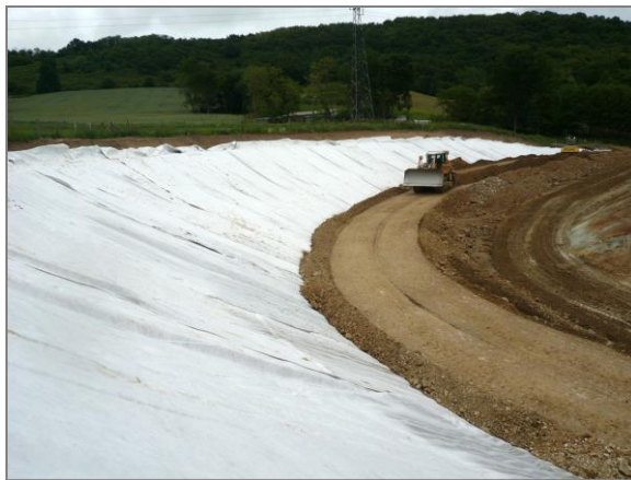
Figures 16: Backfilling – Draining mask and MSE wall
