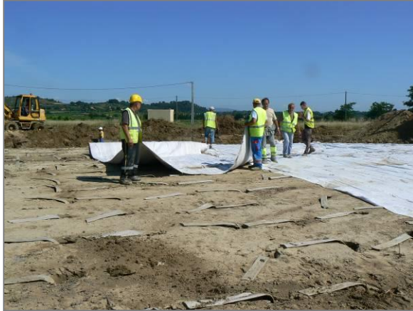
Figures 4: DRAINTUBE® placement over vertical wick drains
