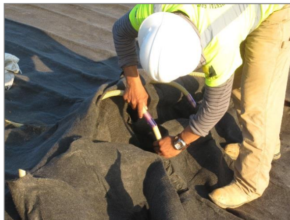
Figure 7: Mini-pipe junction with couplers
