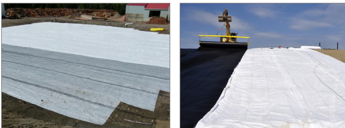
Figures 14: Upper geosynthetic layer placement
