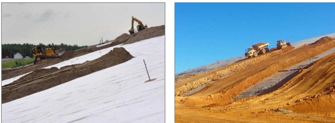
Figures 15: Backfilling
