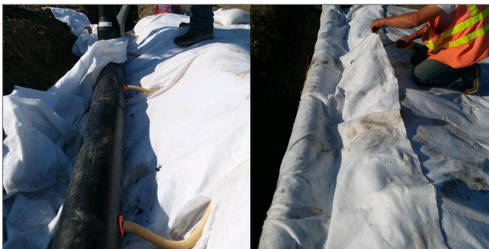
Figures 13: Connection to a plain drain with Quick Connect
