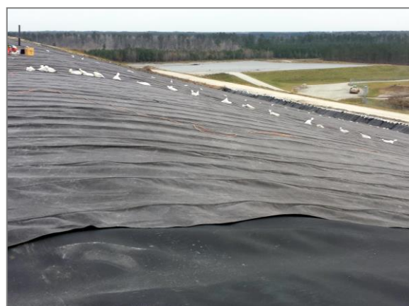
Figure 4: DRAINTUBE® installation
