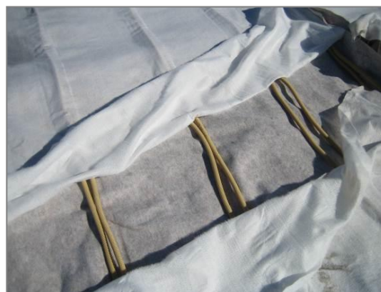
Figures 5: Transverse connections without couplers
