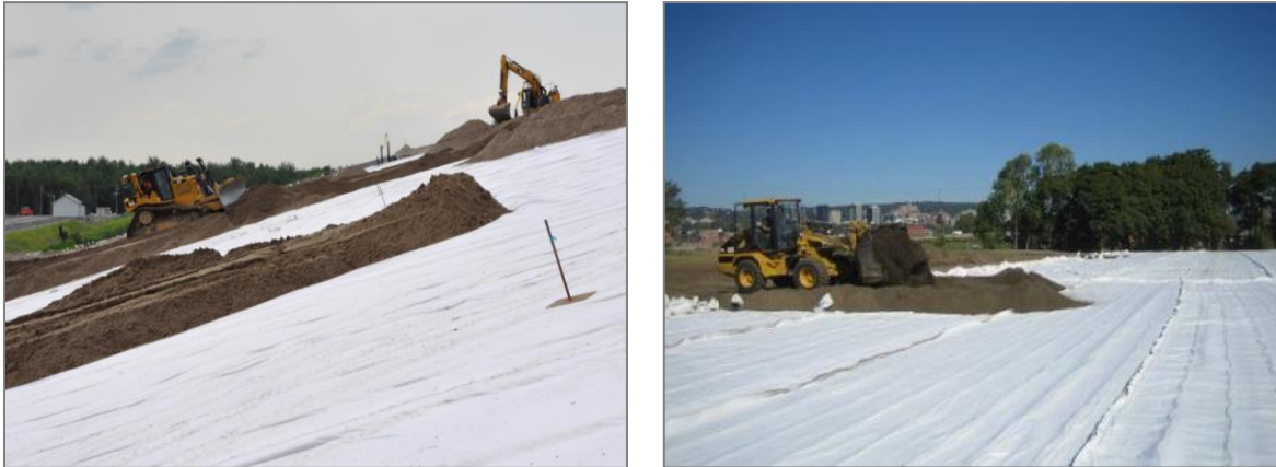
Figures 14: Backfilling
