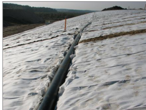
Figure 12: Connection to a plain drain with Quick Connect
