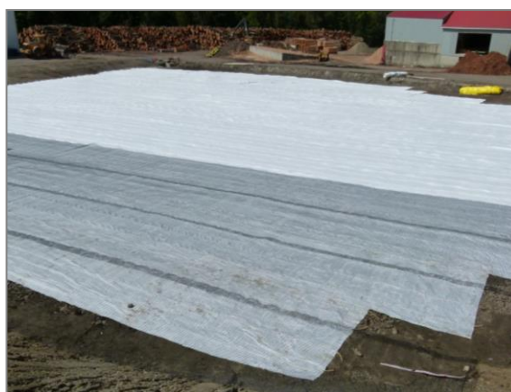
Figure 13: Upper geosynthetic layer placement
