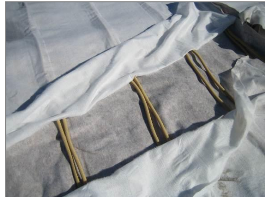
Figures 5: Transverse connections without couplers
