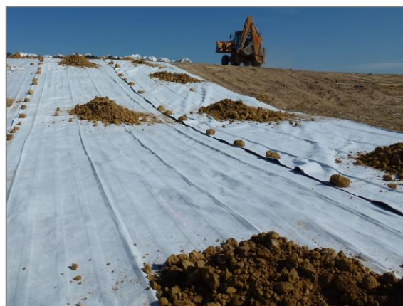
Figure 4: DRAINTUBE ® FTP installation
